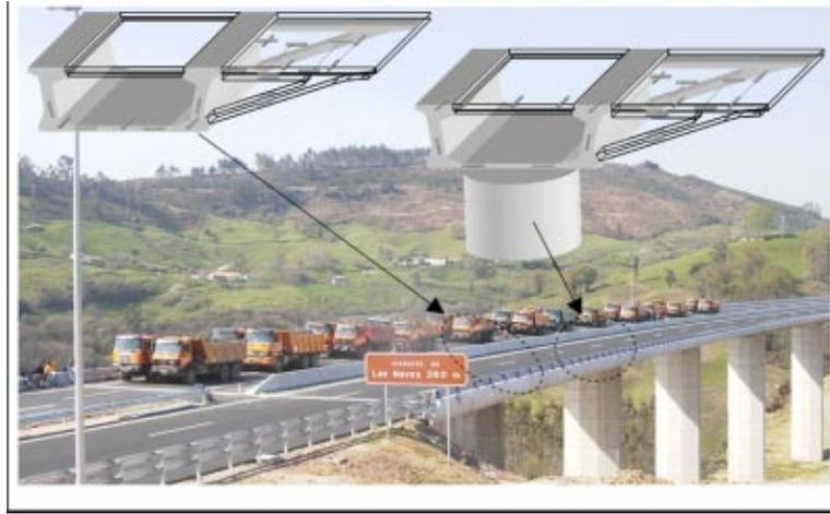
**Fig. 9** Photograph of the monitored structure during the load test. The insets show diagrams of the distribution of transducers in two sections of the bridge.
