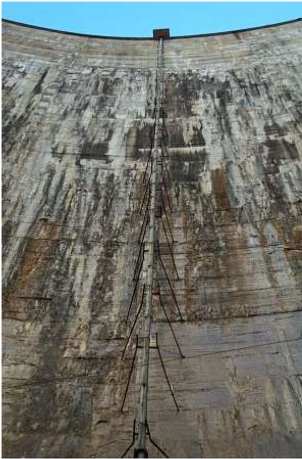
Figure 2. Pendulum in La Cohilla Dam.
