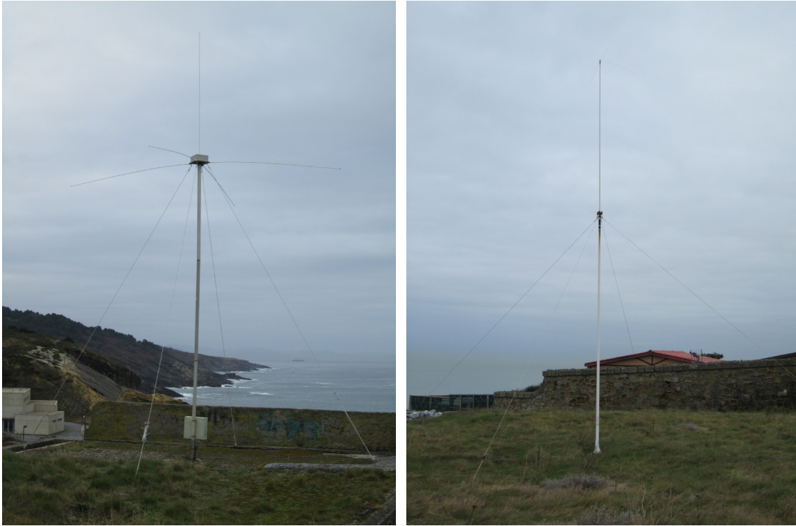
Figure 16: Higer station antennae: (Left) receiver antenna. (Right) transmitter antenna (courtesy of Valentín Urgoiti).
