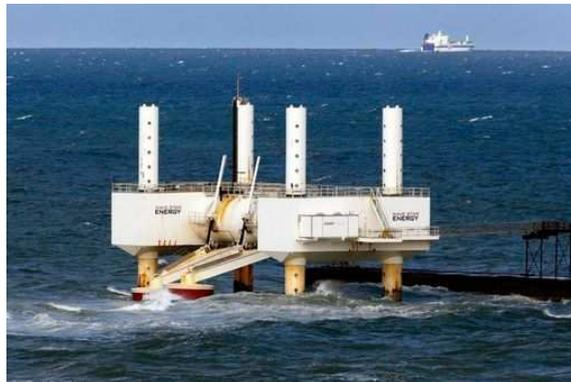
**Figure 2.7:** Wavestar 120 kW in Hanstolm (Denmark)
