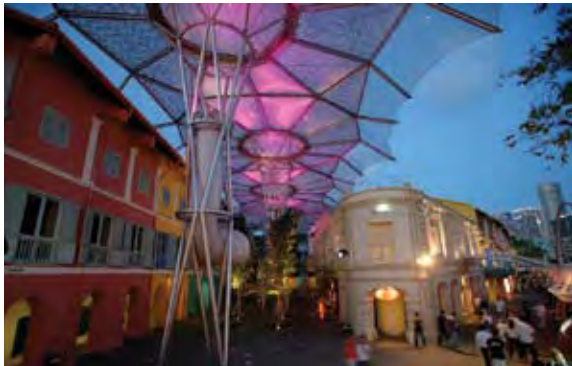
Clarke Quay, Singapore Contractor: Hightex GmbH
