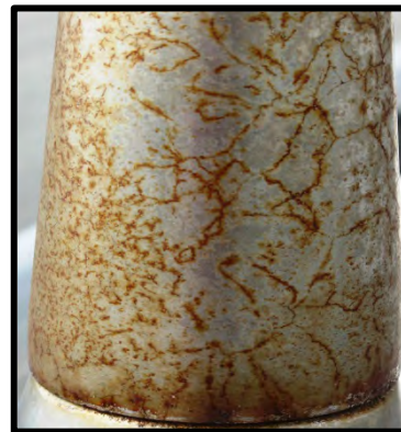
Figure 1: a) Las Llamas Bridge b) lock cover with pitting attack
