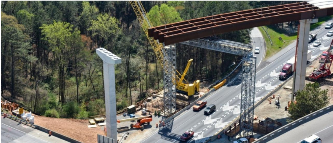
Figure 7. Acrow bridge support system in Atlanta's Northwest Corridor Project [9]
