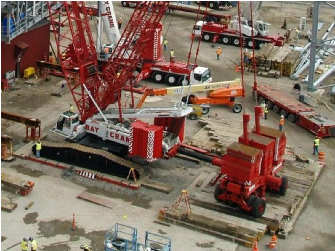
Figure 12. Crane on timber mats
