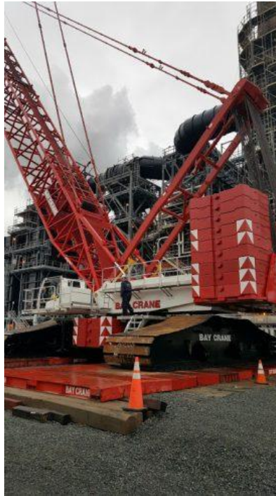
Figure 13. Crawler crane over steel mat
