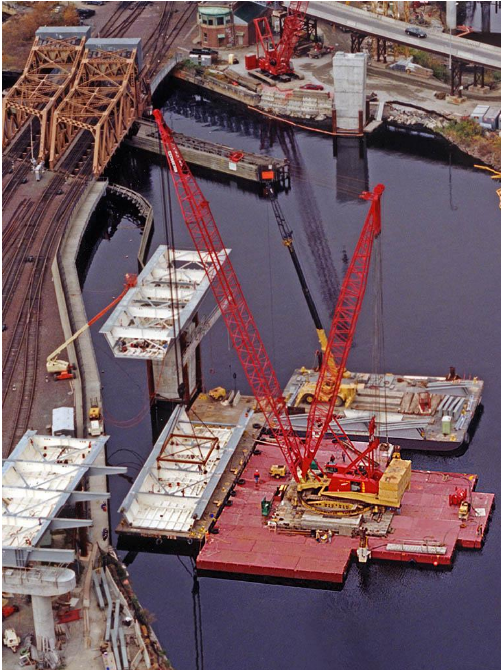
Figure 14. Crane over barge at Big Box Bridge in Boston
