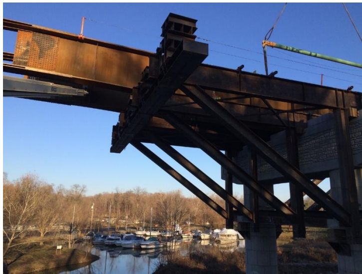
Figure 8. Temporary shoring bracket at Harrod's Creek KY Project [10]
