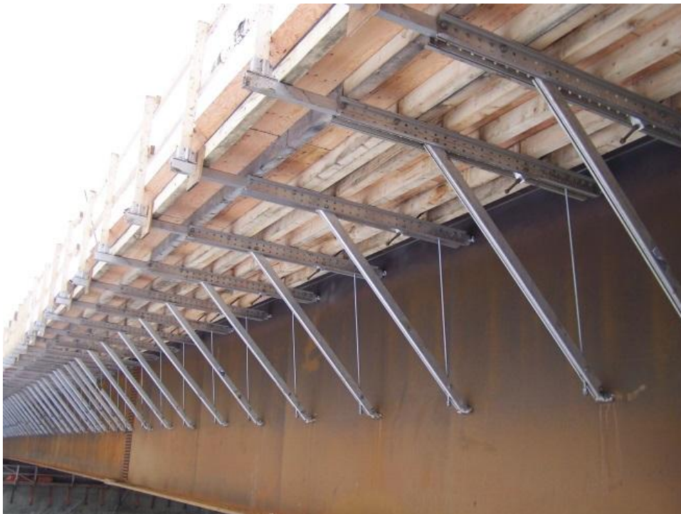
Figure 4. Overhang bracket formwork at steel girder
