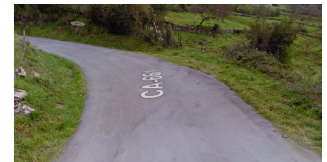
Figure 5.2: Absence of beaconing in curves
