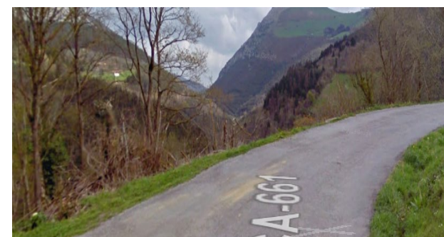
Figure 5.1: Absence of beaconing in curves.
