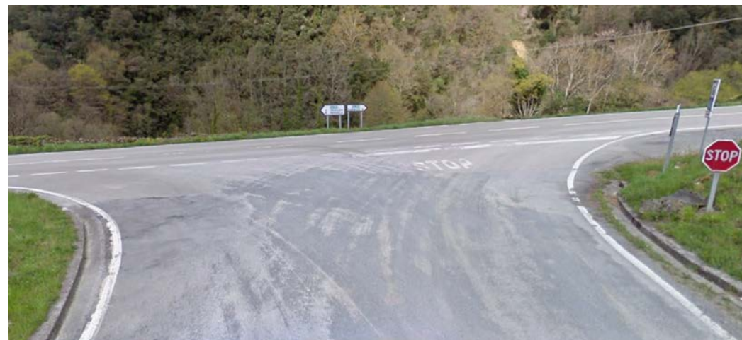
Figure 1: Entrance to the road with poor signaling.
