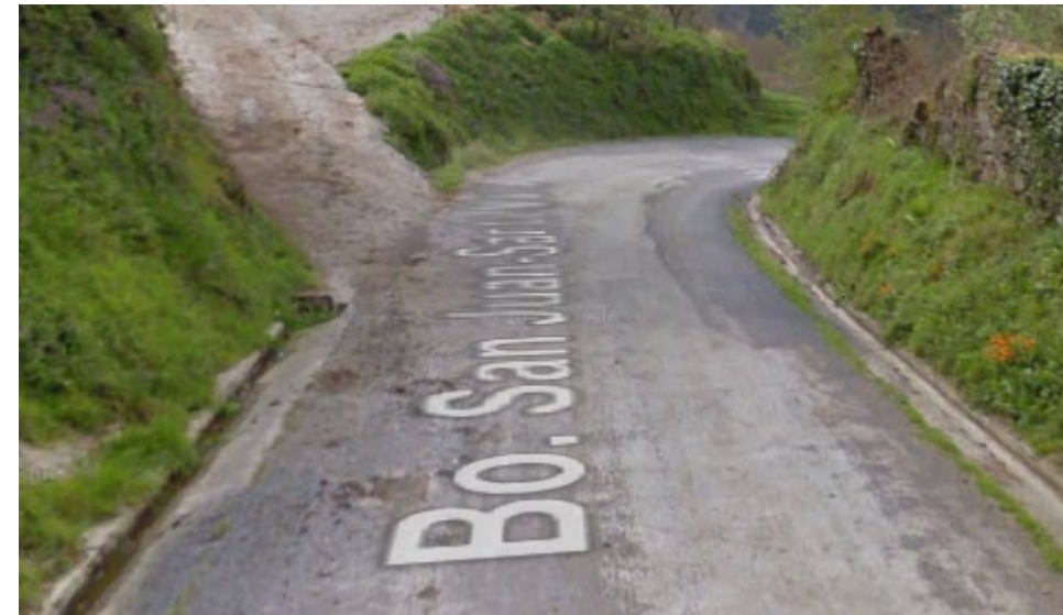
Figure 8: Access to and from homes is unmarked and has poor visibility.
