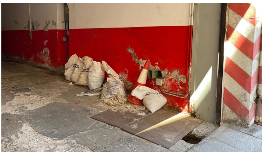
FIGURE R1.7. Presence of dampness in buildings
