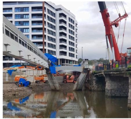
b: Construction process. Longitudinal Rib placement.
