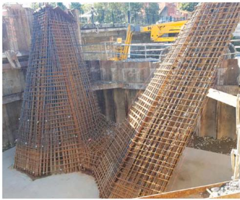
a: Construction process. V shape Pier reinforcement.
