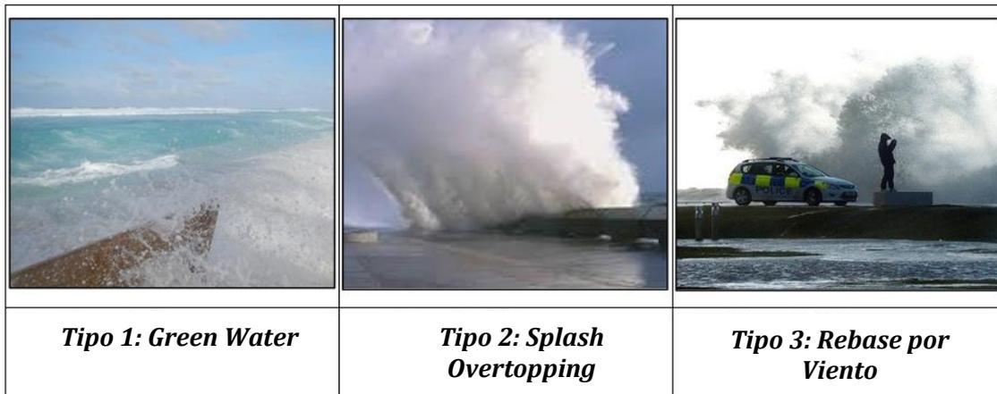
Ilustración 3-48. Tipos de Rebase. [Fuente: (Effect of the overhang length of a recurve seawall in reducing wave overtopping, 2016)]
