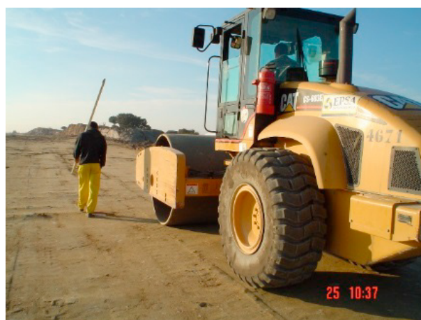
Figure 3. Topographic settlement control after roller pass
