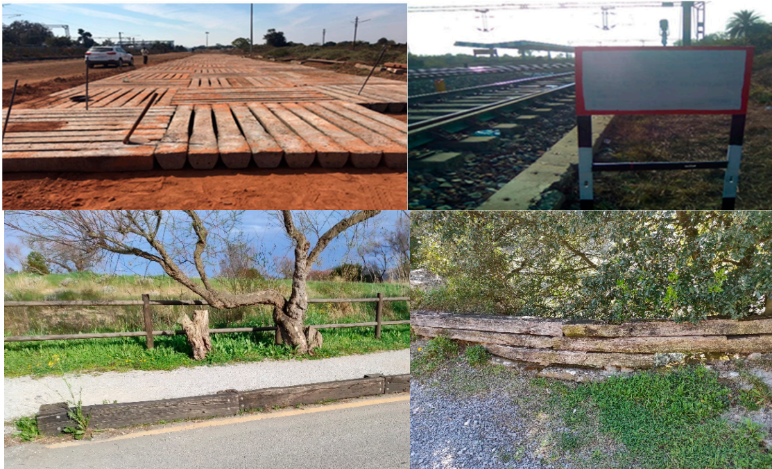
Figure 6. Sleepers are used for making platforms at goods loading areas ( top left ) that are accessible by both road and rail. Ballast alignment along sloped areas of the track to avoid ballast movement ( top right ). Roadsides to separate pedestrian areas ( bottom left ). Pathway sides ( bottom right ).
