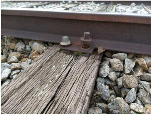
FIGURE 31 Bolts out of place.
