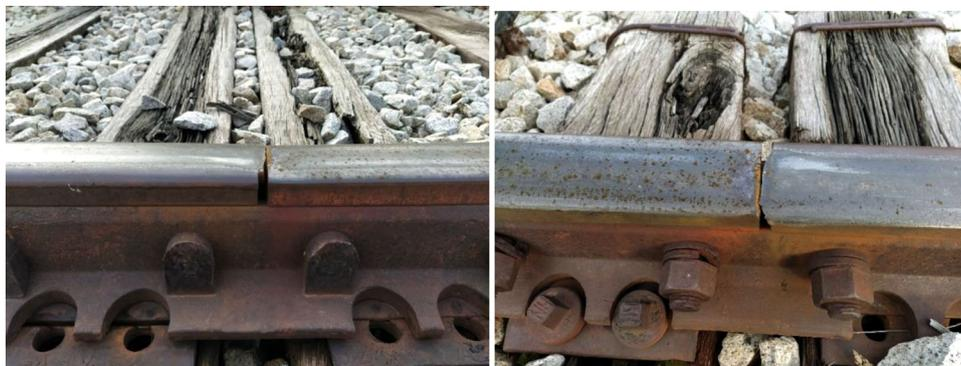
**FIGURE 20** Rail with flange joint without welding, confirmed during visual inspection.
