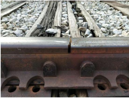
FIGURE 28 Poor condition of junctions with flange joint.
