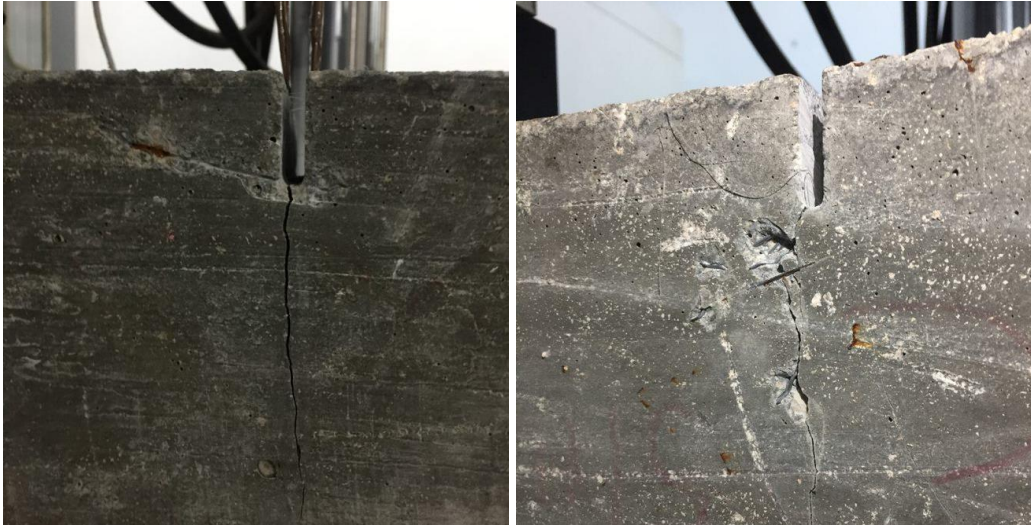
Fig. 31. Cracking of concrete in the fatigue test.
