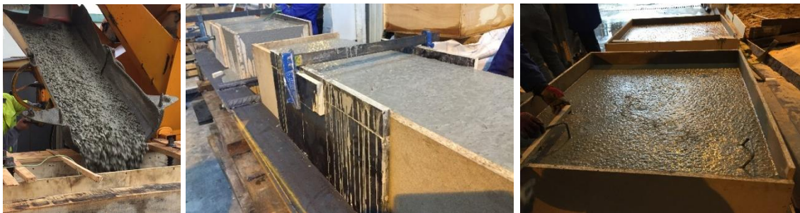
Fig. 5. Concrete pouring (left), BV (centre) and BH (right).
