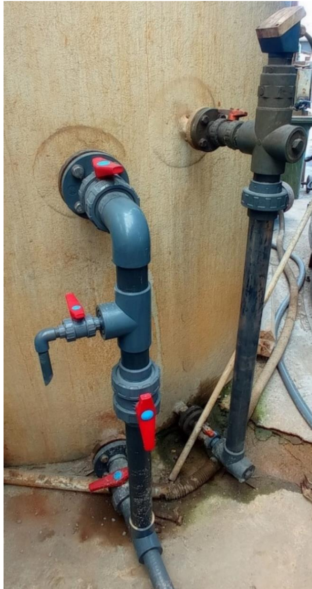
Figure 15. Liquid level and fittings such as valves and piping of the scrubber system.
