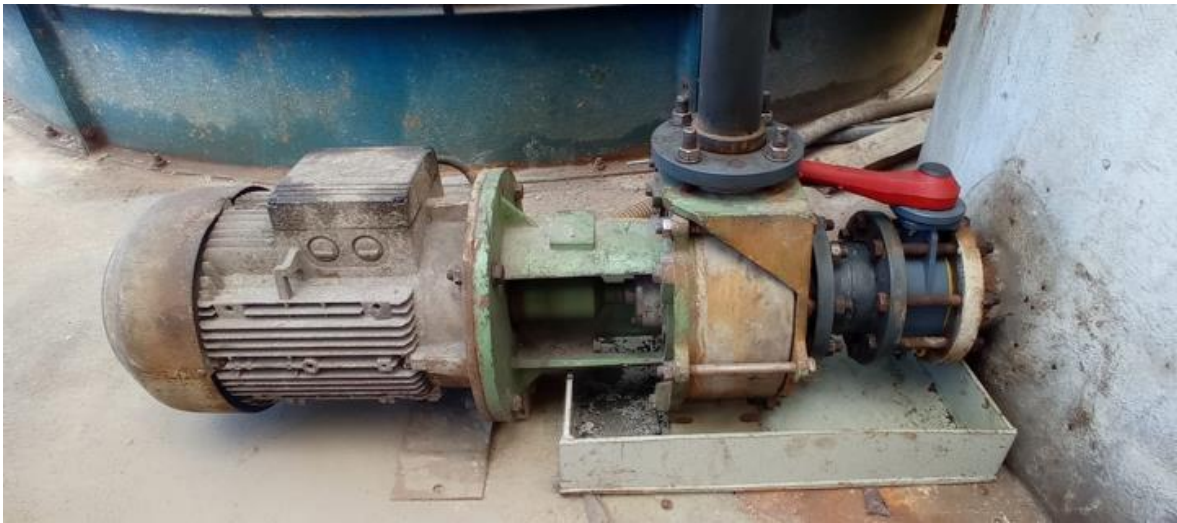
Figure 10. Centrifugal pump of the scrubber system.
