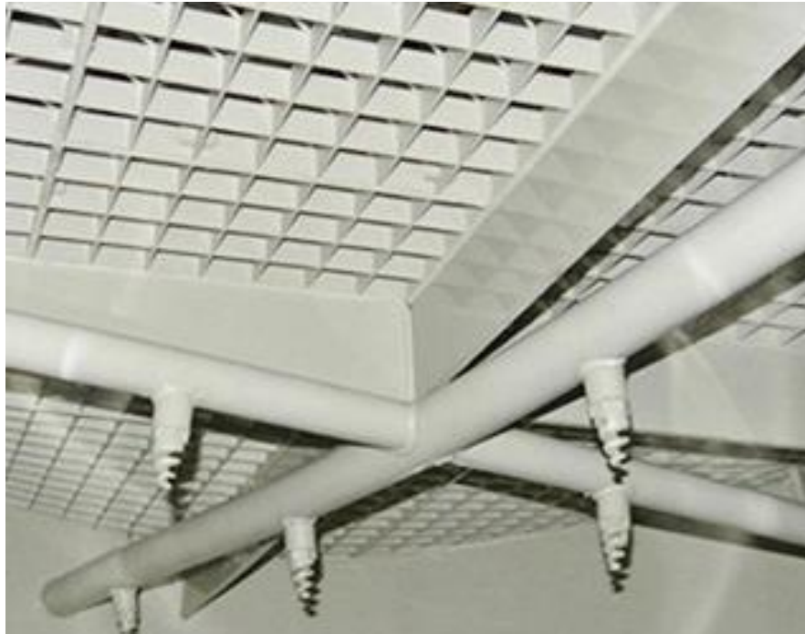
Figure 14. Full cone sprayer of the scrubber system.
