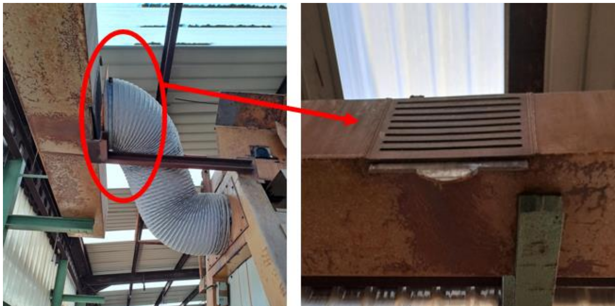
Figure 8. Side extraction system for capturing gases during the pickling process.
