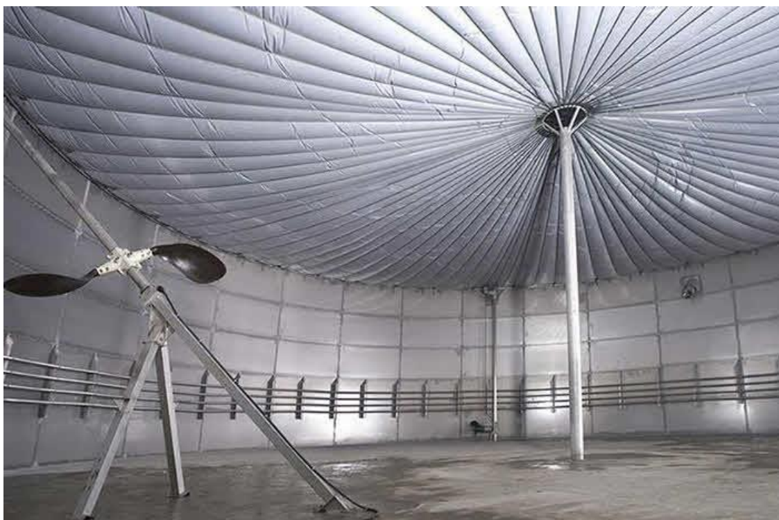
Figura 4.6 Interior Biodigestor (WELTEC Biopower)
