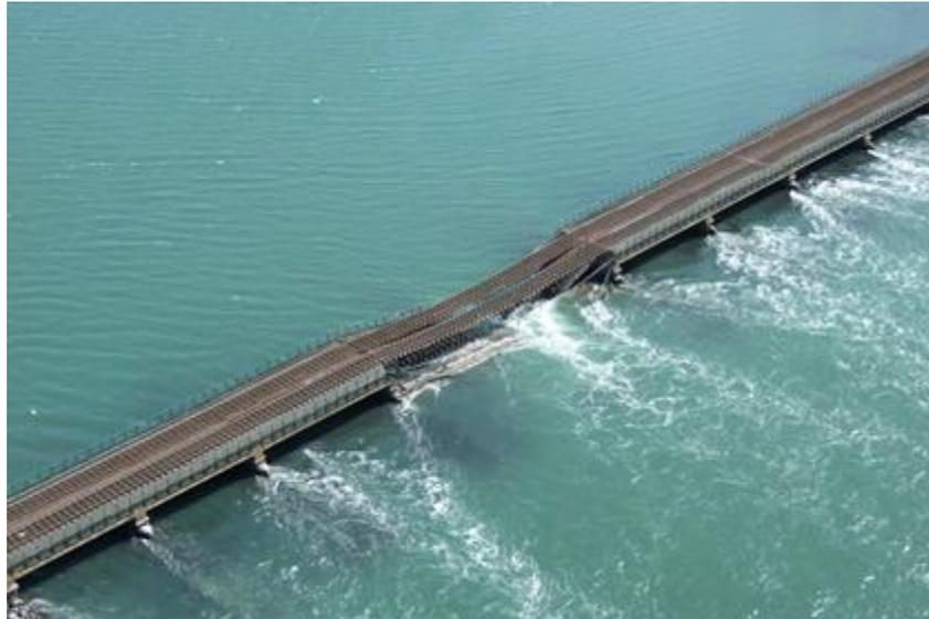
*Figure 2: Railway bridge collapse in Ireland caused by scour undermining in piers. Image from <https://www.newcivilengineer.com/scour-revealed-as-cause-of-irish-bridge-collapse/5207460.article>*
