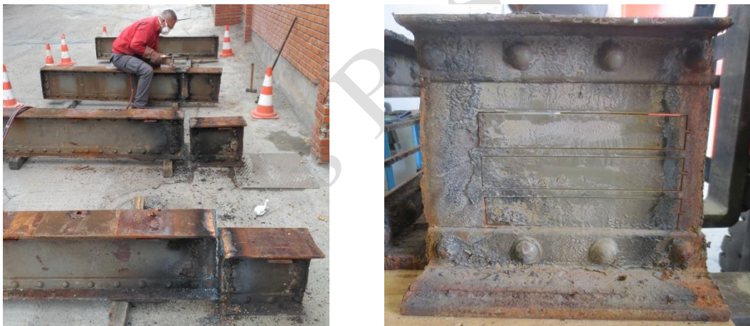
Figure 2. Puddle iron plates cut from the web of riveted stringers of Redondela bridge.
