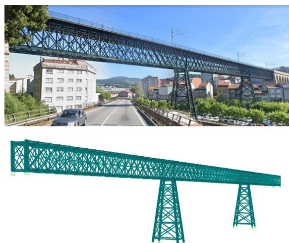
Figure 3. General view of Redondela Bridge and 3D numerical model using SAP2000® software.
