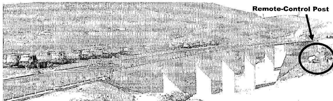
Figure 8. Photograph of a remote sensing during the load test
