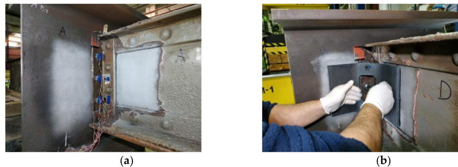
Figure 23. Installation of CFRP angles on the connection. (a) Metal surface preparation. (b) CFRP adhesive bonding.
