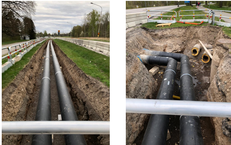
Figure 29: Piping system for District Heating in Linköping
