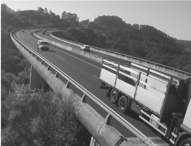
Figure 7 Vehicle detection example over pier 1
