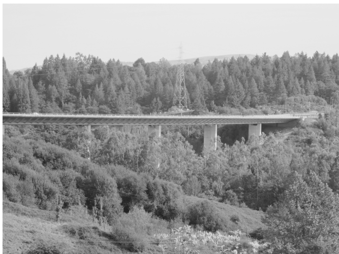
Figure 1 Las Navas bridge A8 highway (Spain)
