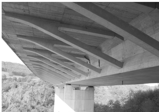
Figure 2 Bracing beams from Las Navas bridge
