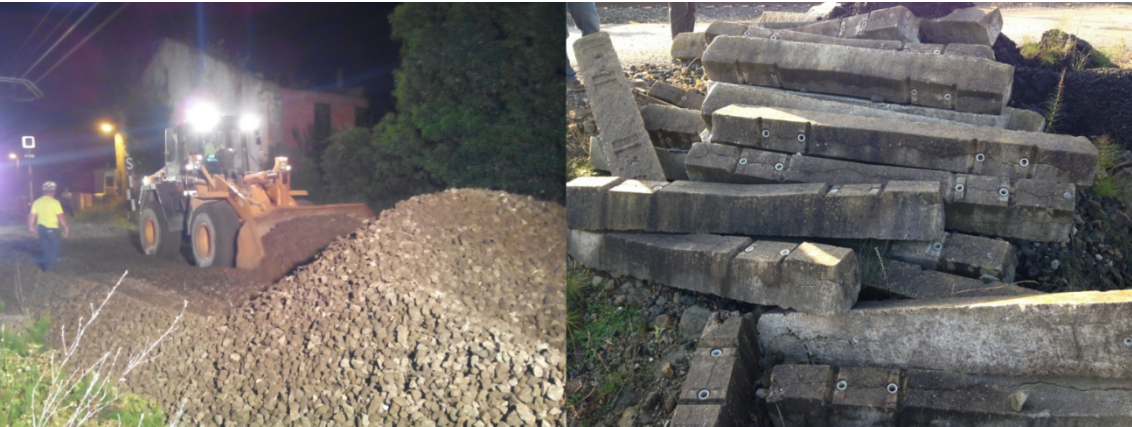
Figure 1: Ballast waste generation in the renewal of ballast track (left) and out-of-use concrete sleepers (right).
