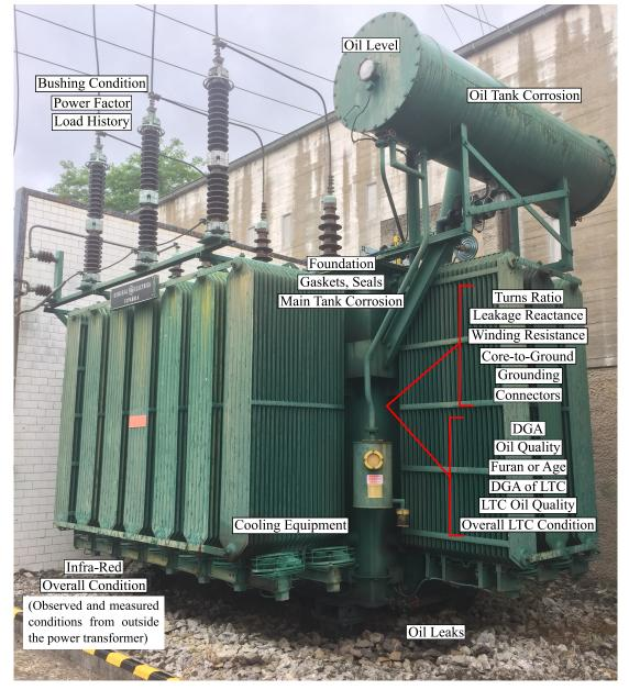
Figure 2. Location of the parameters measured for the HI calculation of the transformer.
