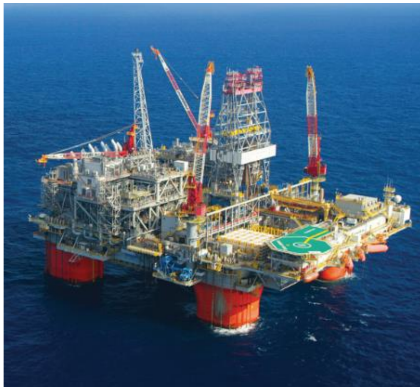
Figura 38: Plataforma semi-sumergible BP Thunder Horse [23]
