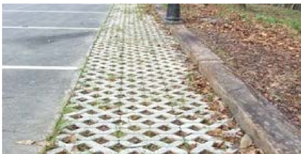
Figure 6. Filter drain with concrete reinforced cells surface
