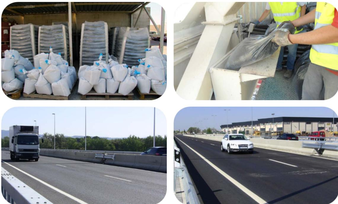
Figure 47. Construction process and final pilot road of mixtures modified with polymeric waste
