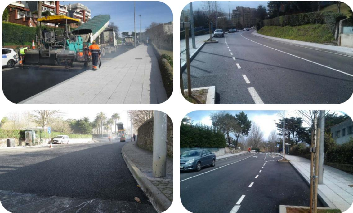
Figure 45. Construction process and final mixtures of the experimental pilot road
