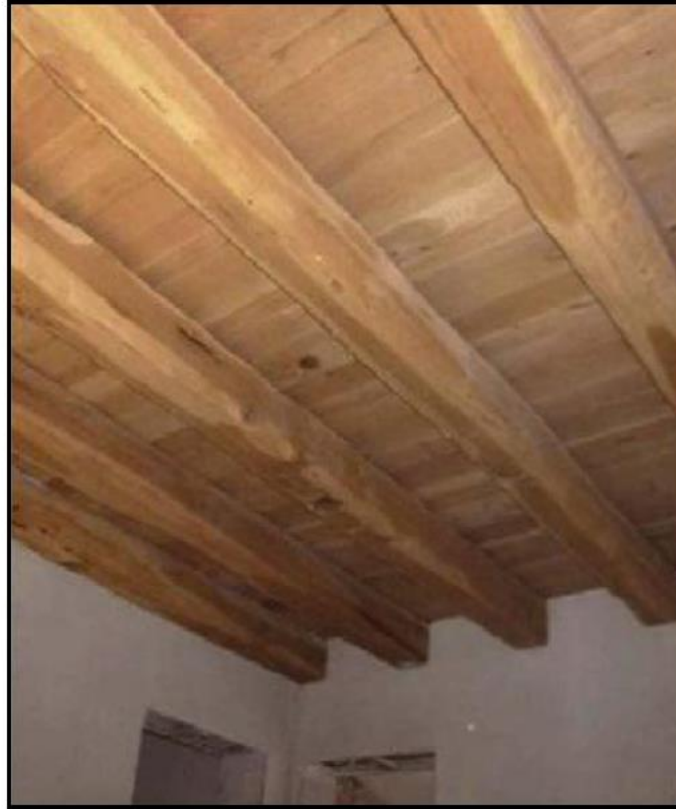
Figure 8 An example of Molfetta's typical ceiling/roof structure [12]
