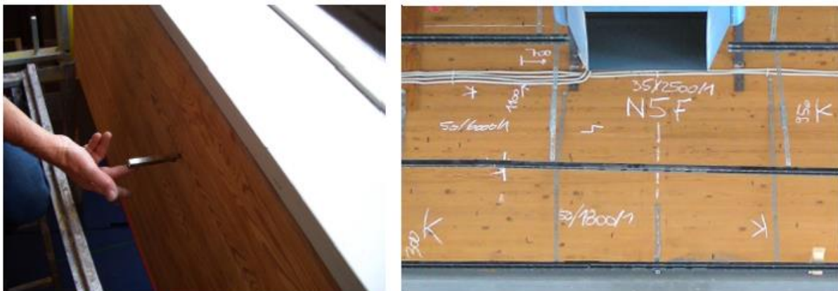
Figure 6 - Example of Crack Measuring; Example of Crack Mapping (Dietsch, Philipp, & Heinrich, 2011).
