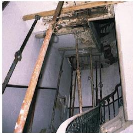
Figure 1 – Rotten Timber Structure with Safety Propping (Cruz, et al., 2015).
