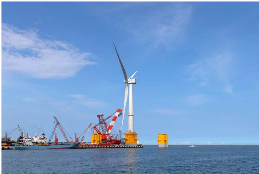
*Figure 11: The 7MW floating wind turbine by Fukushima FORWARD consortium (courtesy of consortium).*
